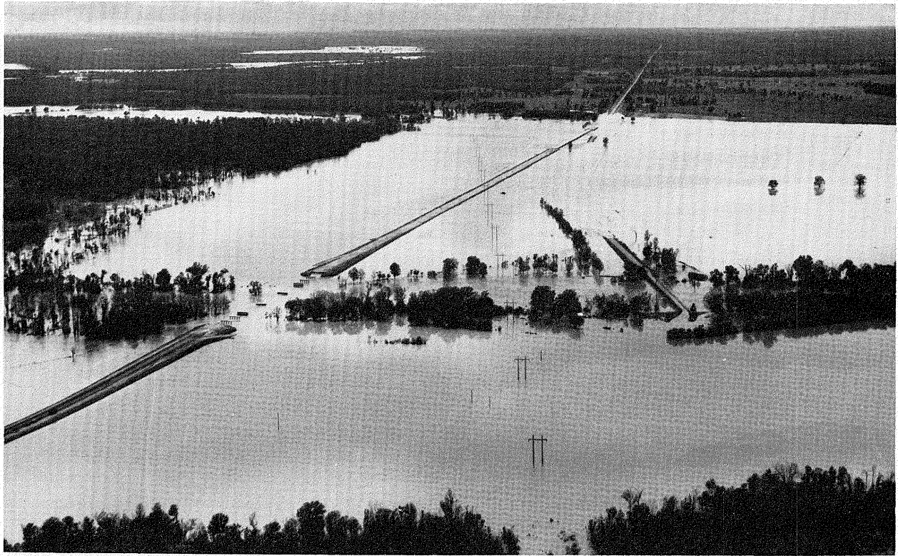
PLATE 7A.—Trinity River, west of Crockett, Tex., May 1, 1957. Approaches to highway bridge flooded, also river-bottom grazing land. (Official photo—Corps of Engineers, Fort Worth District.)
