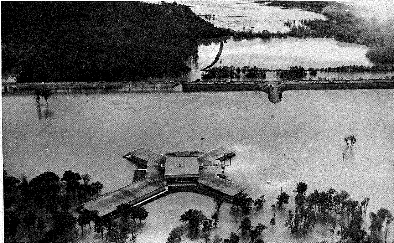
PLATE 6B.—Trinity River, about 8 miles downstream from Commerce Street Bridge, Dallas, Tex., April 25, 1957, stage 34 feet. (Crest 39.7 feet on April 27.) View shows Country Club grounds downstream from the Dallas Floodway Levee. (Official photo—Corps of Engineers, Fort Worth District.)
