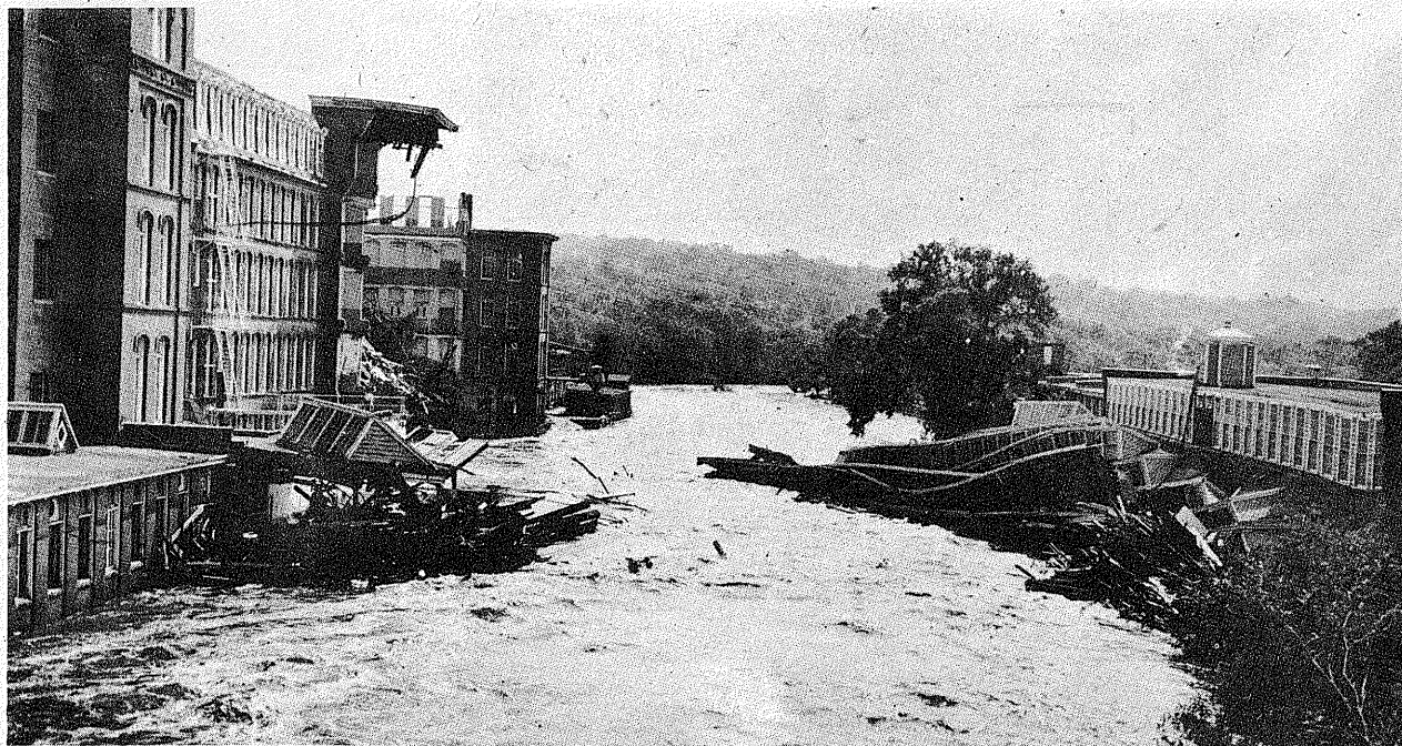
PLATE 4A.—Blackstone River at Manville, R. I. Scene showing extensive damage to the Atlantic Mills and the Royal Electric Co. (Photo courtesy Army Engineer Corps.)
