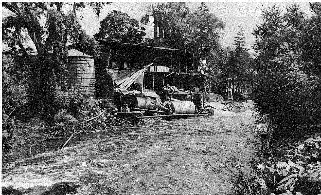
PLATE 4B.—Quinebaug River at Southbridge, Mass. Scene showing sheared off section of the Ames Textile Corporation Mill. (Photo courtesy Army Engineer Corps.)
