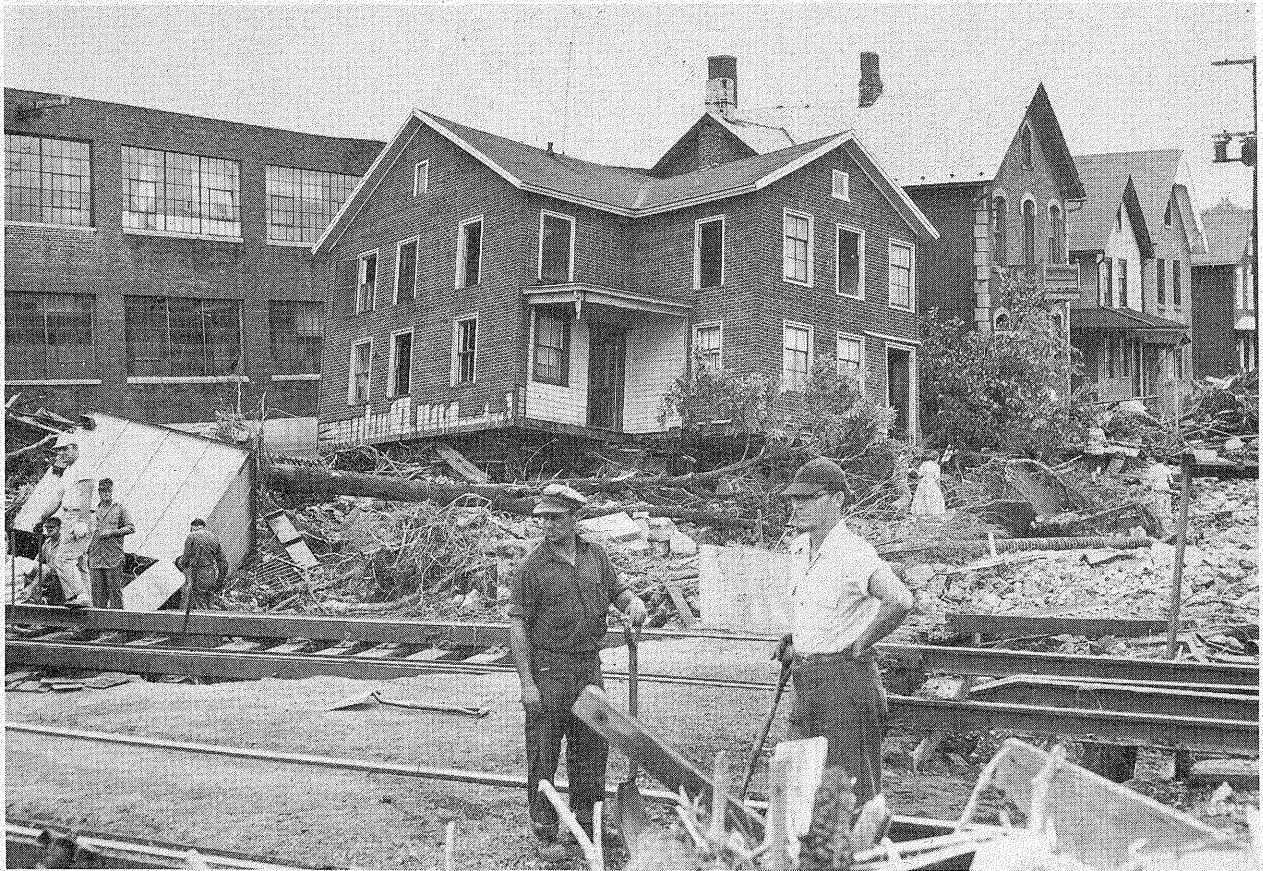
PLATE 8B.—Damaged homes and railroad bed, South Scranton, Pa. (Photo courtesy Pennsylvania Department of Highways.)
