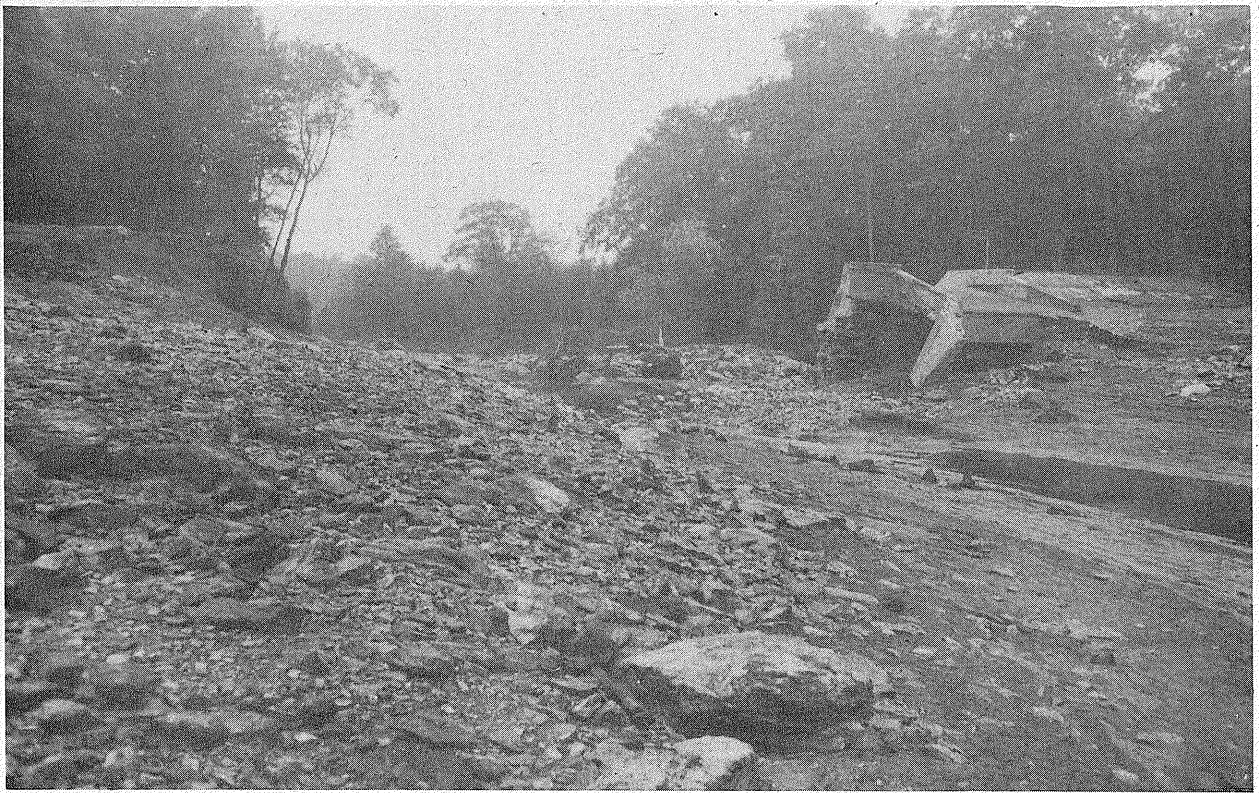
PLATE 6A.—Charlton, Mass. Scene showing dam failure at Glen Echo.
