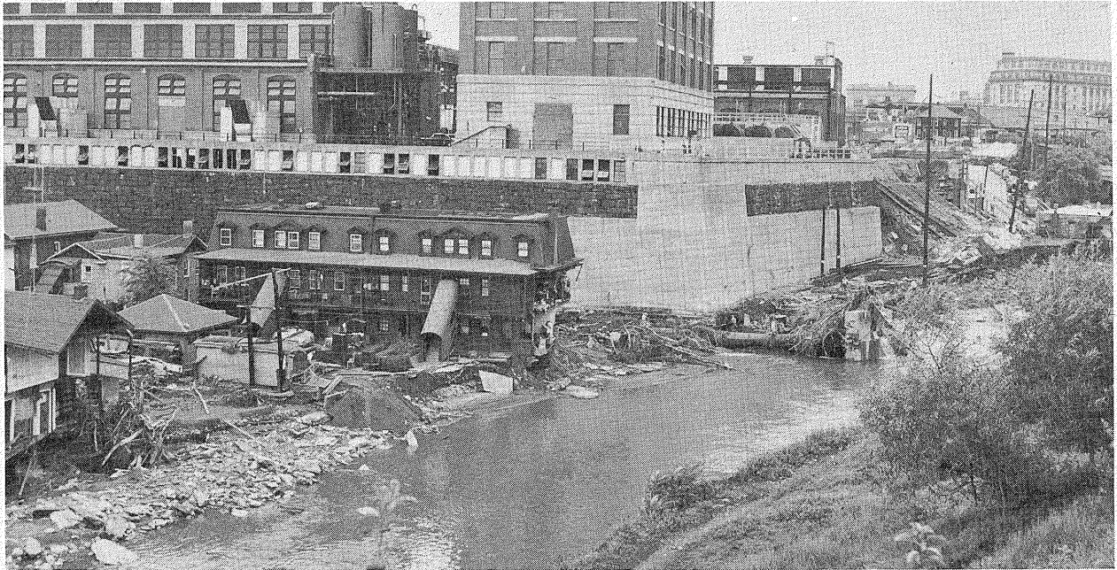
PLATE 8A.—Damage caused by flooding Roaring Brook at Scranton, Pa. (Photo courtesy Pennsylvania Department of Highways.)
