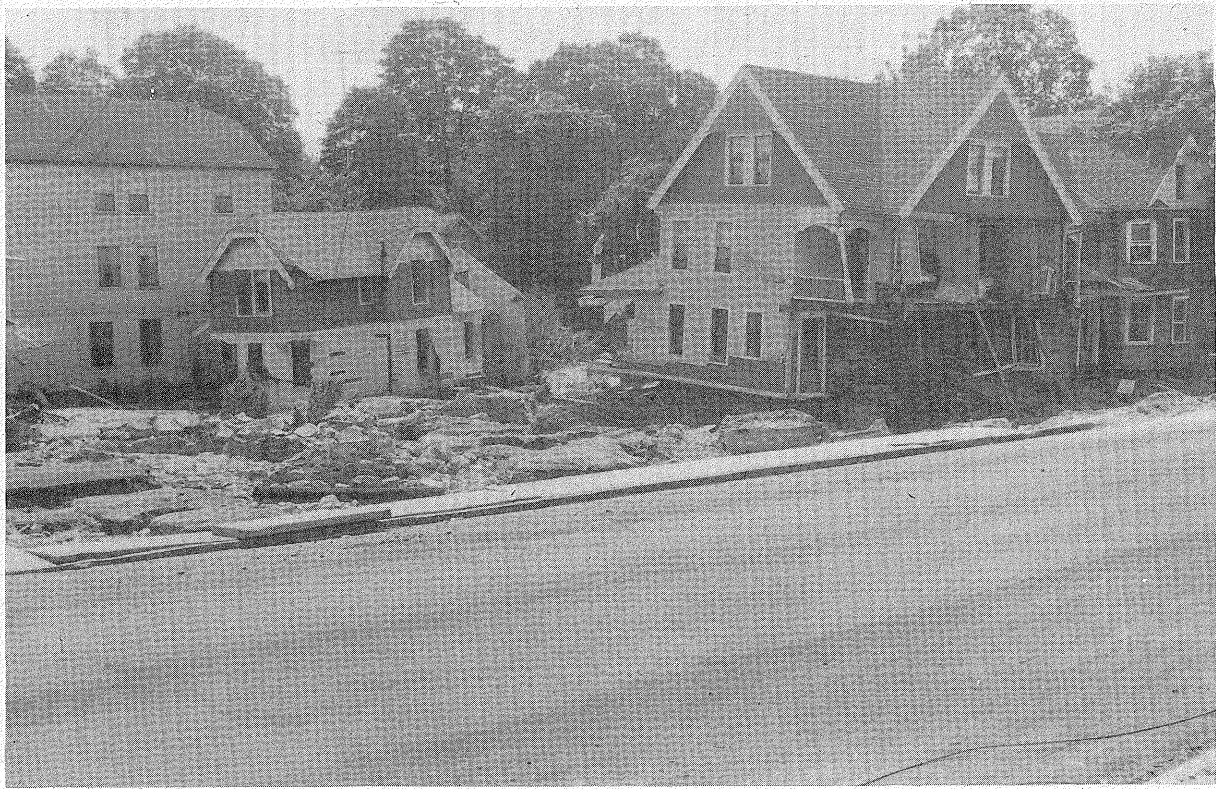
PLATE 3A.—Naugatuck, Conn. Scene of residential damage along Naugatuck River.
