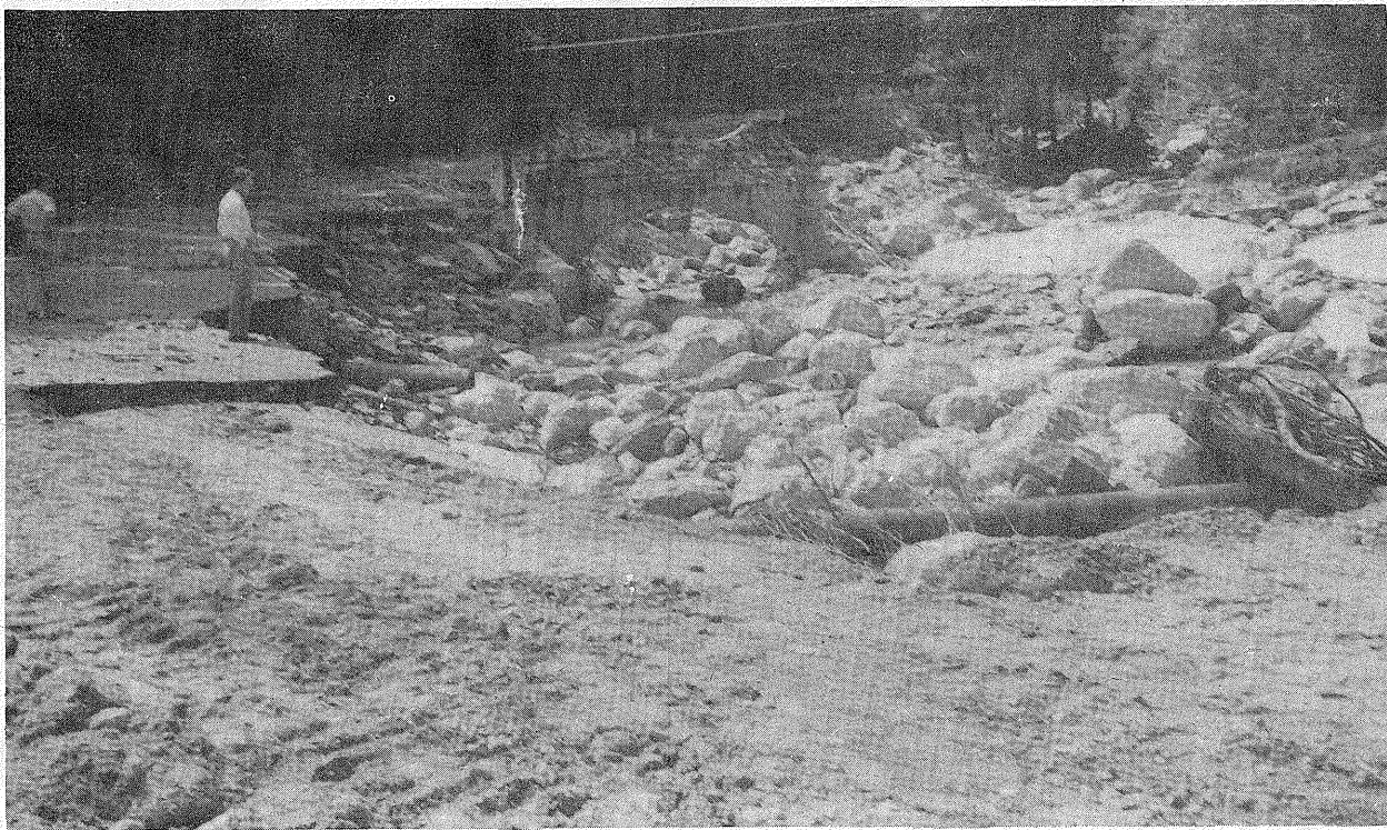
PLATE 5B.—Westfield, Mass. Scene showing road damage east of Westfield.
