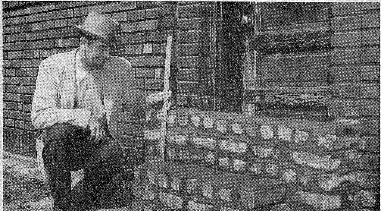
B. Dubuque, Iowa, April 17, 1952. City garage was ready for the crest 8 days before it arrived. Present stage was 19.6 feet and crest was 22.7 feet on April 25. Note stone masonry protection. ( Courtesy Mel Schieltz, Telegraph Herald. )
