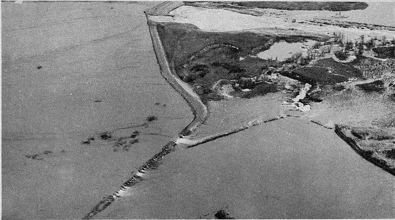
A. Frenchman Dam, Valletown, Mont. View at 2 p. m., April 15, 1952. Dikes overflowing in foreground. ( Official photo U. S. Corps of Engineers. )
