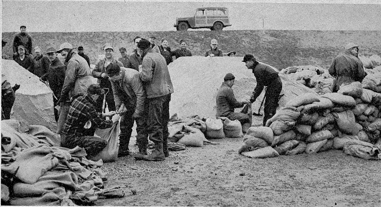
A. Flood fight behind the levee, 60th and Walker Streets, North Omaha, Nebr. Workers at this and other sites filled sandbags at the rate of 15,000 an hour. About 5½ million bags were used. (Courtesy Omaha World Herald.)
