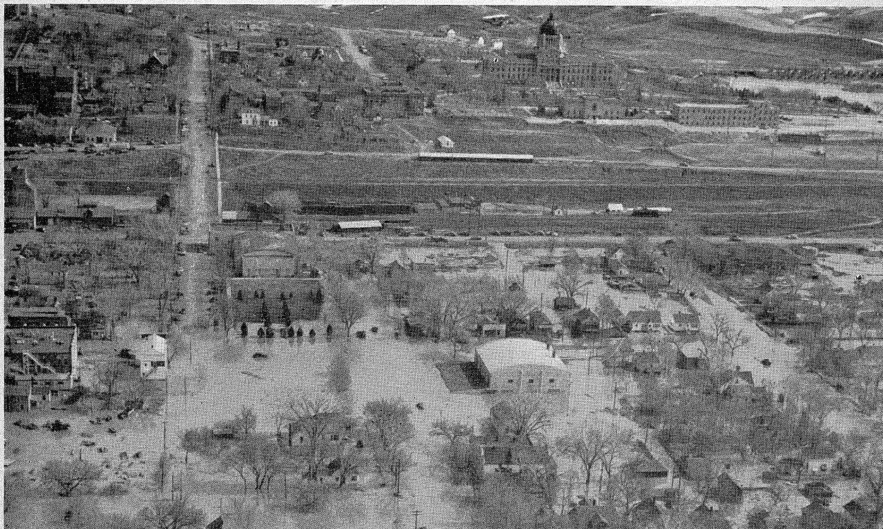
B. Pierre, S. Dak., looking across town toward Capitol Building. One hundred blocks inundated. Photo taken Thursday noon, April 10, 1952, shortly before the river reached its crest of 25.35 feet.
