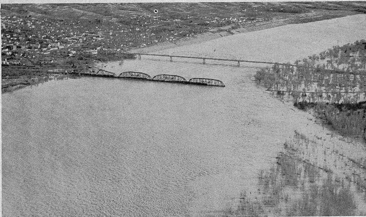
A. Missouri River at Chamberlain, S. Dak. Note railroad cars on bridge in foreground, placed there to keep rest of span from moving out. April 1952.
