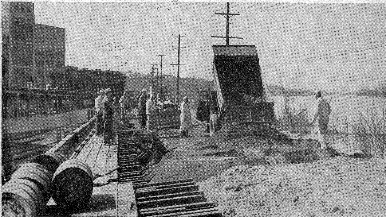
B. Mississippi River at South St. Paul, Minn., stage 22.1 feet, April 16, 1952. Emergency levees protecting meatpacking companies. (Official photo U. S. Corps of Engineers.)
